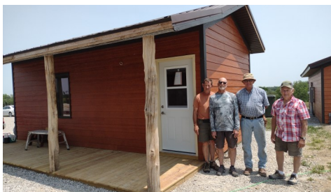
Volunteers standing by 1 of the 2 cabins completed just in time for summer camps!
